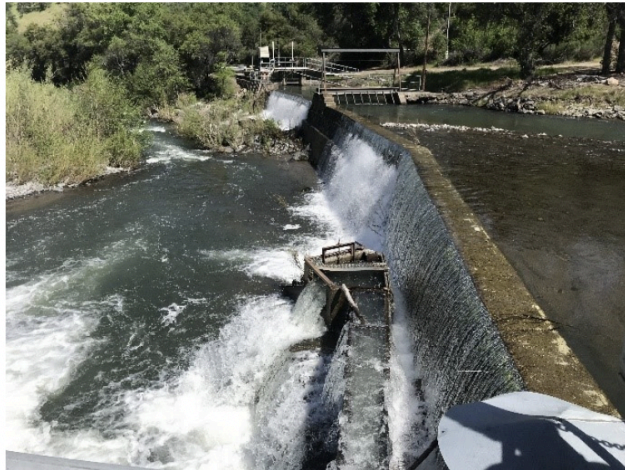
Coleman Diversion Dam on South Fork Battle Creek Photo: California Water Boards
